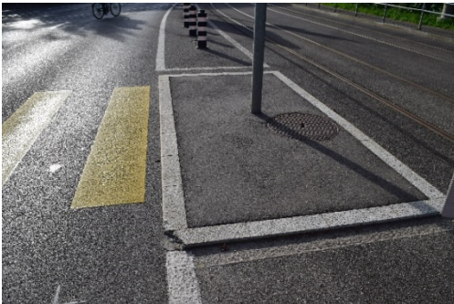
Defekte Randabschlüsse
